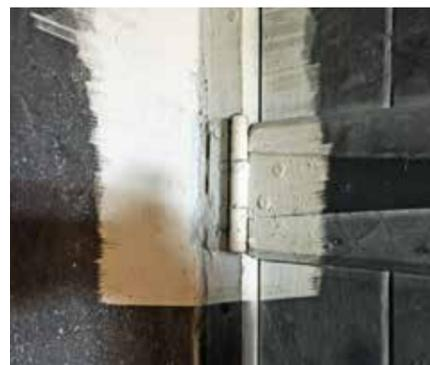
Figure 3: The laser beam was reflected off the white plaster boards and white painted walls, while at the same time removing the soot.
