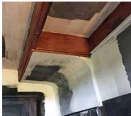
Figure 1: Saving the ceiling battens
